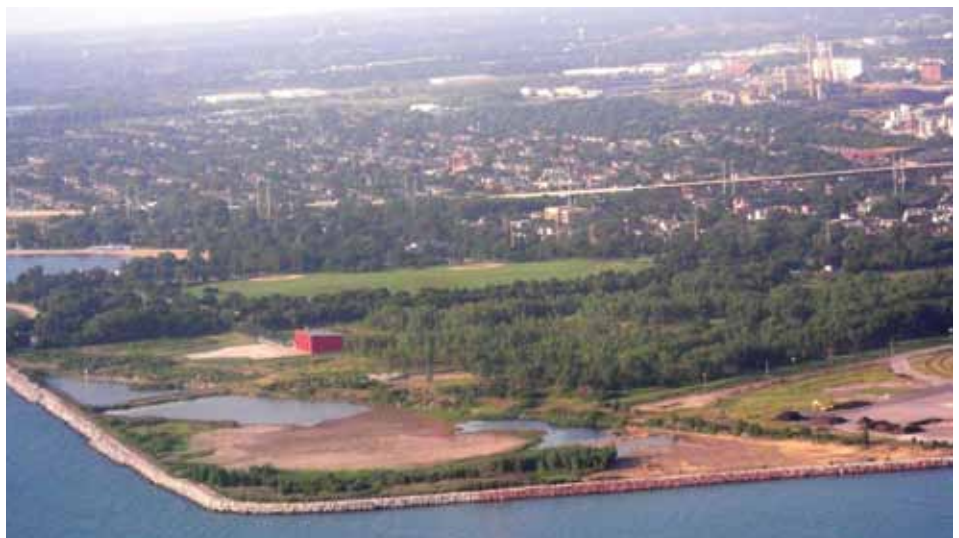
The Confined Disposal Facility is the triangle-shaped concrete bathtub filled with toxic material from the Calumet River. The aerial photo is taken from Lake Michigan looking south to Calumet Park.
