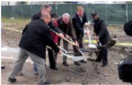
Pictured at Adams and Sangamon (left to right) are Ernest Wong, Architect from Site Design Group, Chris Gent from the Chicago Park District, Beth White from Trust for Public Land, and Aldermen Bob Fioretti (2nd Ward) and Walter Burnett (27th Ward).
