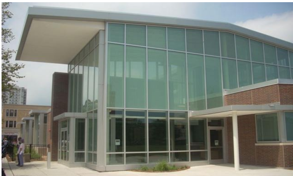
The long-awaited Gale Park Fieldhouse (1610 W. Howard Street) in Rogers Park opened in August and features a fitness center, gymnasium and club house.
