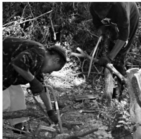
Cajette and Keenan saw buckthorn stakes to help support the terracing.
