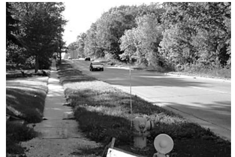
A road widening project in suburban Orland Park may gobble up 1.8 acres of McGinnis Slough Forest Preserve land and reduce the buffer between the slough and the road.
