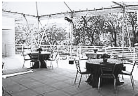
Officials at the Peggy Notebaert Nature Museum wish to enclose its 5,600 square foot second-floor terrace on the building's west side to provide on-site office space, and move the current terrace to the third floor.
